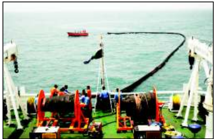
Fig 11. Deployment of boom
