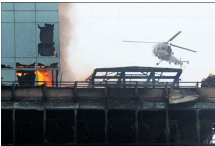
Stranded fire fighters on Top of Lotus Business Park
