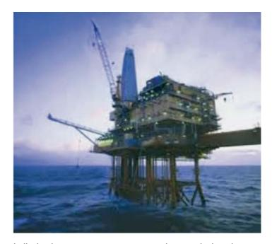
is limited exposure to movement due to wind and water forces. However, these platforms cannot be used in extremely deep water, it simply is not economical to build legs that long.
